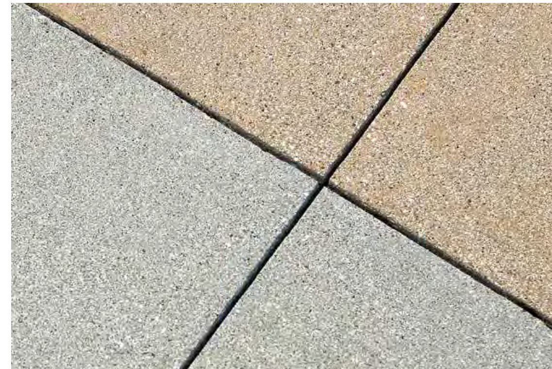
DECORATIVE CONCRETE ACID-ETCH TOPCAST G3 FINISH (ETCHES NEW CONCRETE TO EXPOSE FINE AGGREGATES AND ELIMINATE SHEEN AND CLARE OF NEW PLAIN CONCRETE), AS SHOWN OVER PLAIN AND INTEGRALLY COLORED CONCRETE. ACCENT COLORS TO BE WARM GREY (DAVIS COLOR SEQUOIA SAND OR SIMILAR) AND SOFT GOLD (DAVIS COLOR SPANISH GOLD OR SIMILAR) OR OTHER NEUTRAL COLOR COORDINATING WITH ARCHITECTURAL IMPROVEMENTS.
