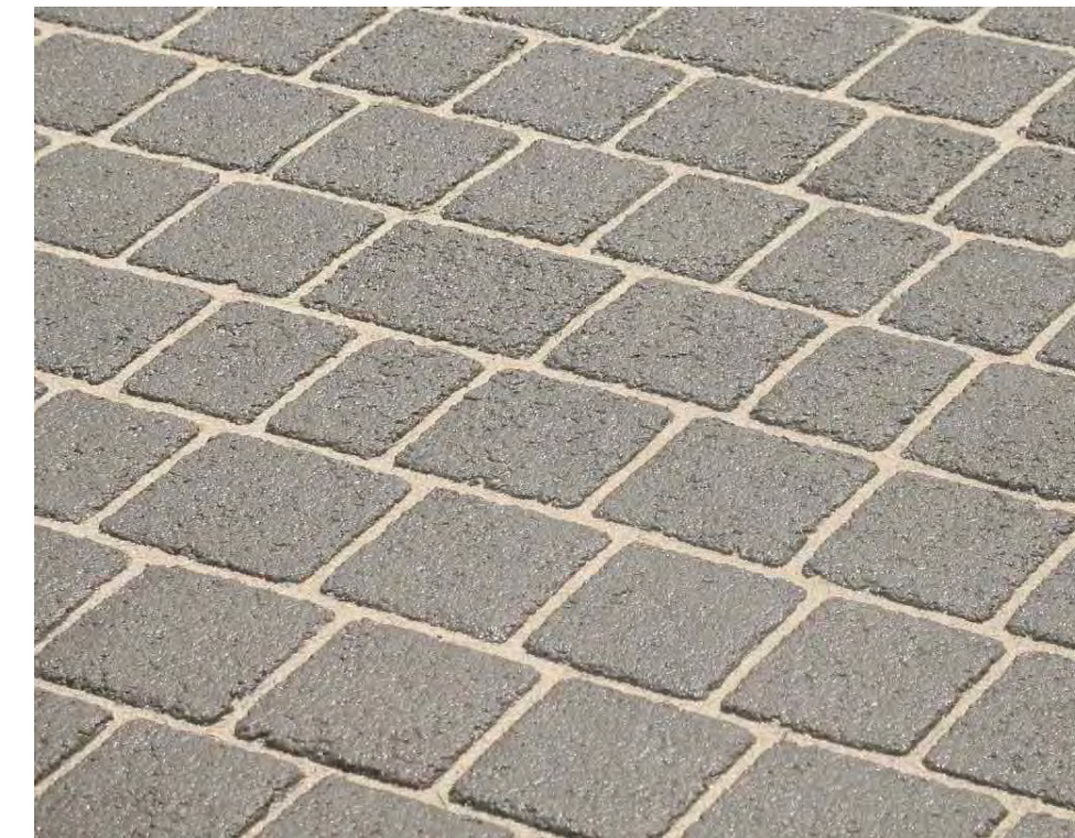
STAMPED ASPHALT (ALTERNATE FOR STAMPED CONCRETE) RANDOM COBBLE, RUNNING BOND (SHOWN WITH STREETBOND COATING WITH CONTRASTING FIELD/GROUT COLORS)
